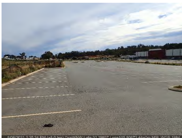
Photo ID: Photo 2 Looking at the bitumen carpark and shops.
