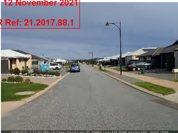
Photo ID: Photo 1 Looking at the road, infrastructure and houses.
