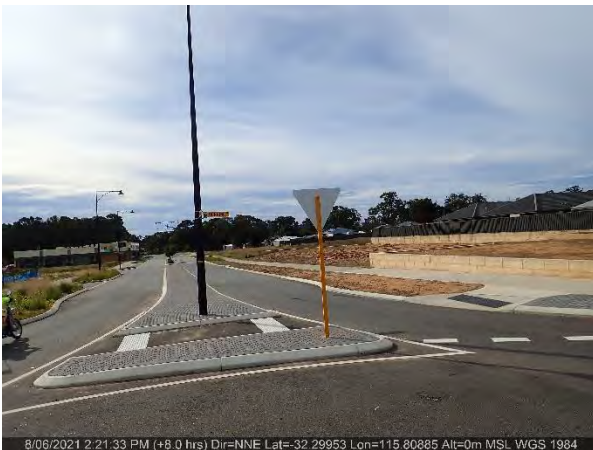
8/06/2021 2:21:33 PM (+8.0 hrs) Dir=NNE Lat=-32.29953 Lon=115.80885 Alt=0m MSL WGS 1984 Photo ID: Photo 11 The bitumen road, road reserve and cleared lots.
