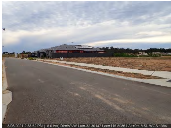
Photo ID: Photo 14 The established infrastructure east of the development site.
